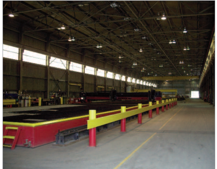
Automated cutting tables in DSR’s massive fabrication building.
